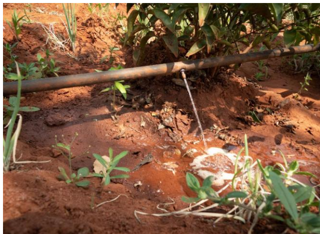
Drip irrigation system.
